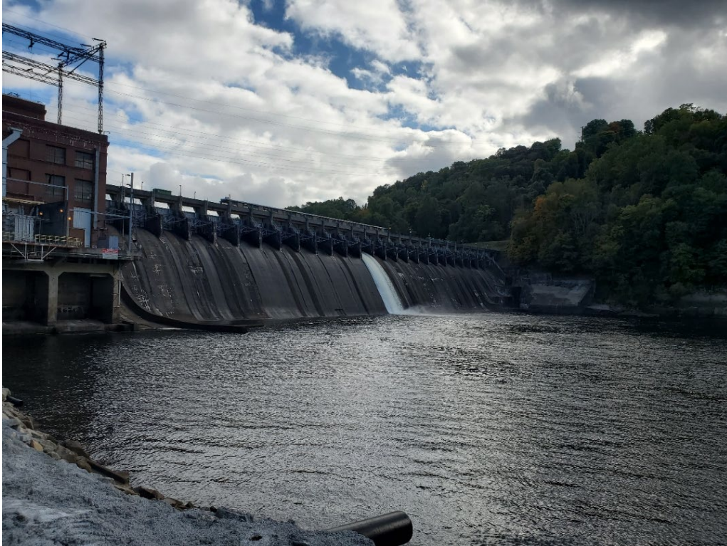
Photo 4.14 View of Project Dam from Tailwater Fishing Pier
