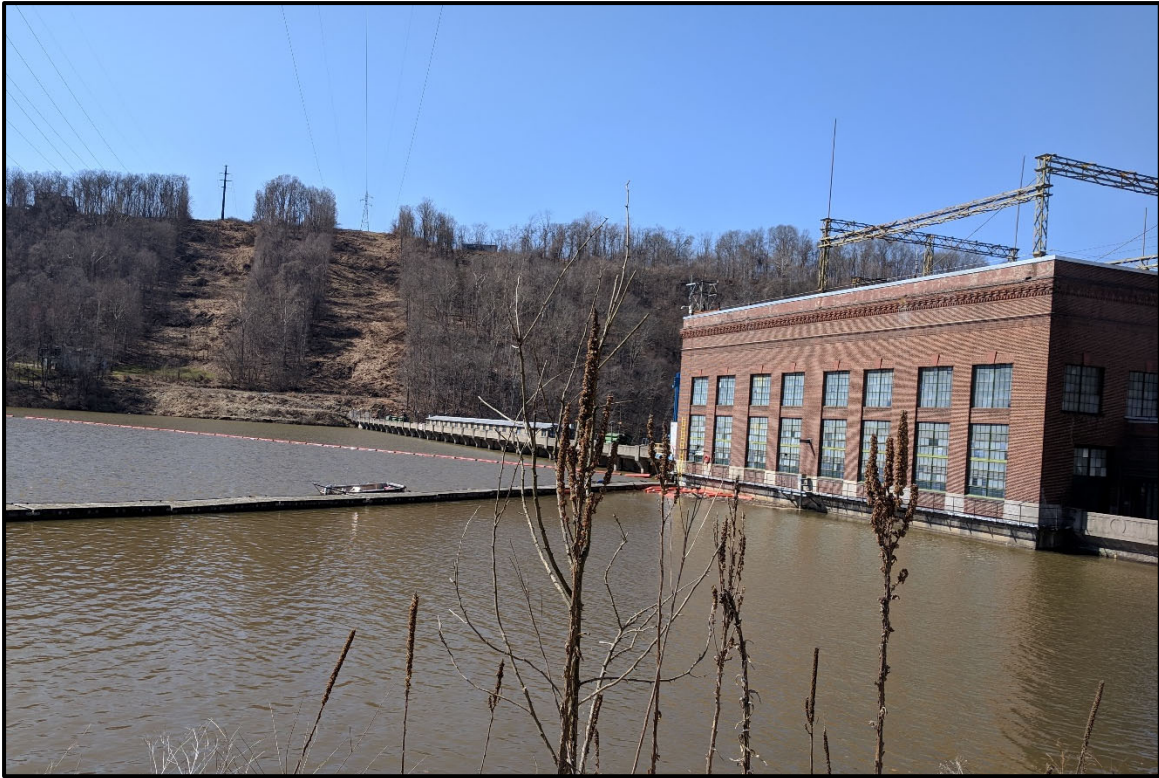
Figure 2. View of Powerhouse and Dam at Lake Lynn Hydroelectric Project.
