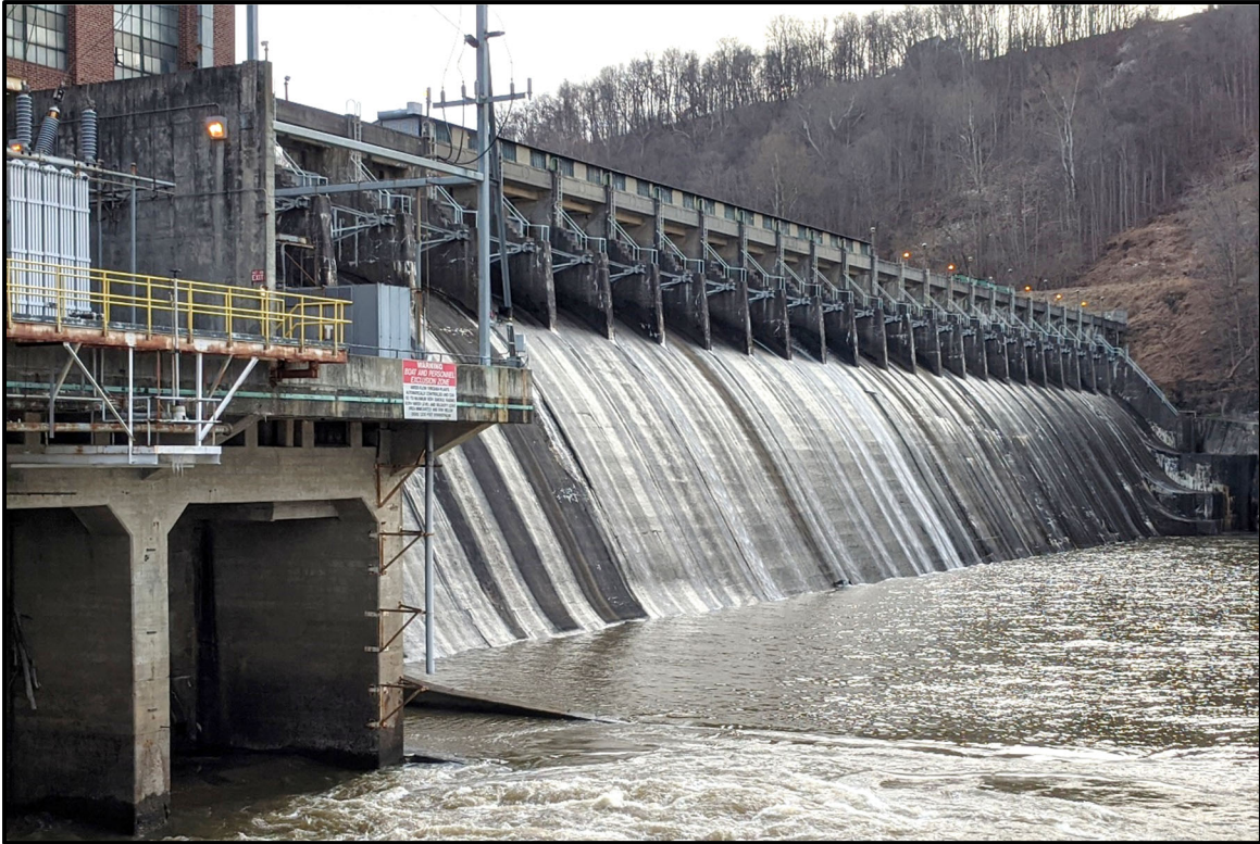
Figure 4. View of Dam at Lake Lynn Hydroelectric Project.
