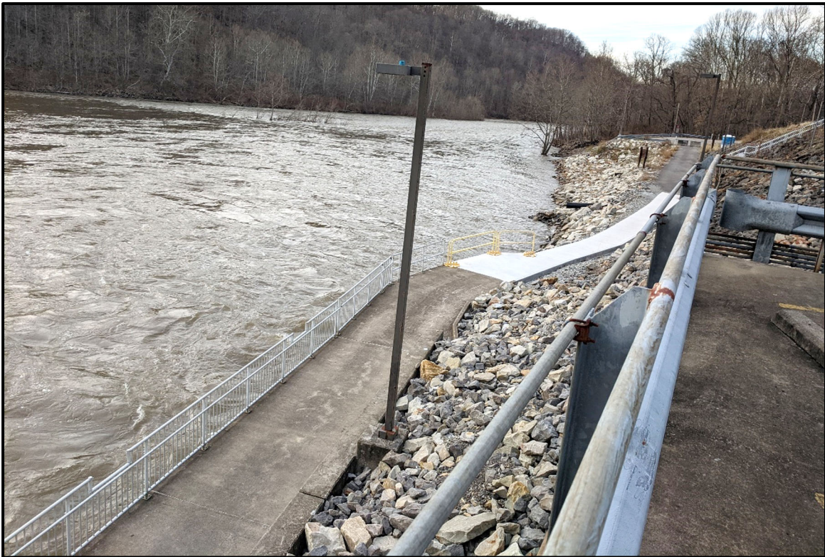
Figure 7. View of Tailrace Fishing Pier at Lake Lynn Hydroelectric Project.
