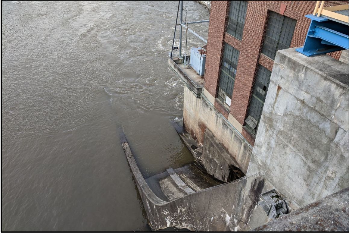
Figure 8. View of Sluice at Lake Lynn Hydroelectric Project.
