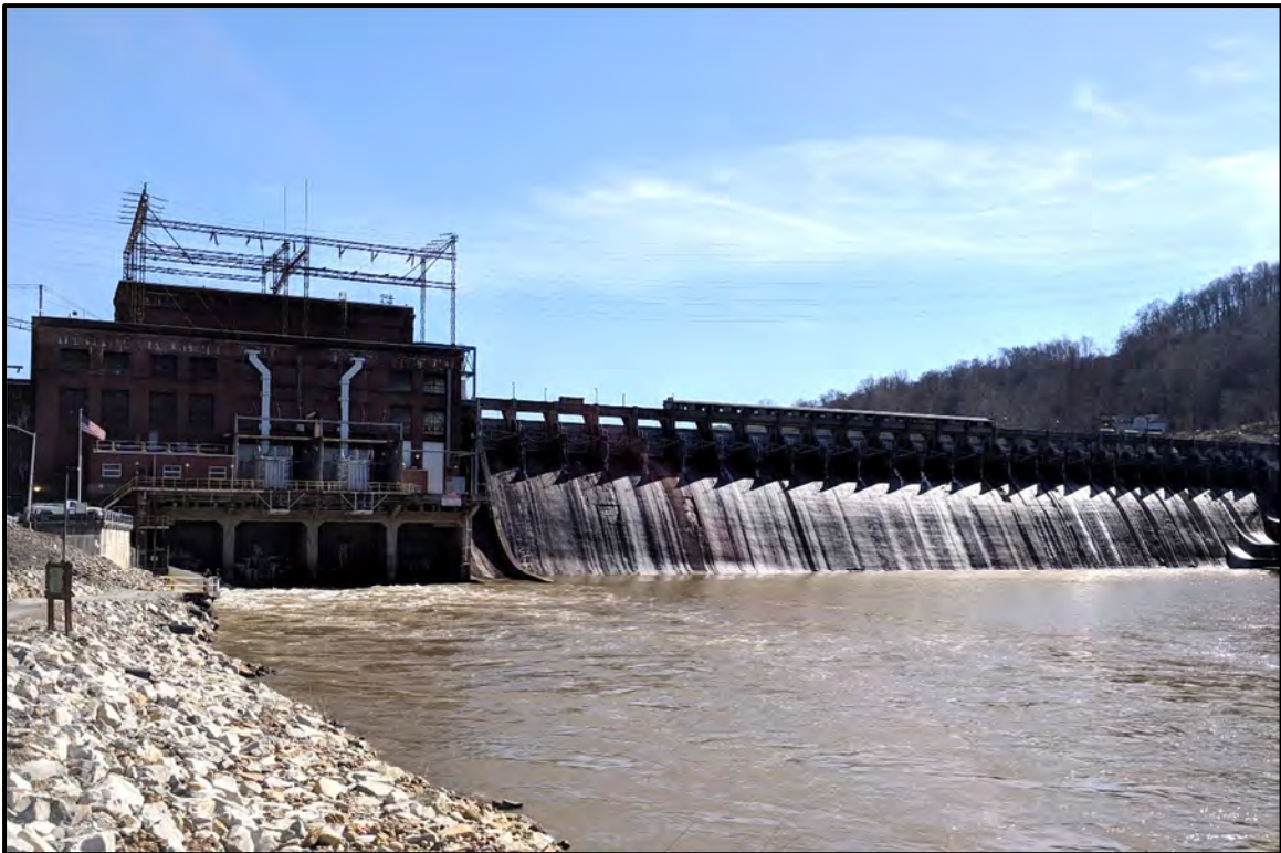
Figure 3. View of Powerhouse and Dam at Lake Lynn Hydroelectric Project.
